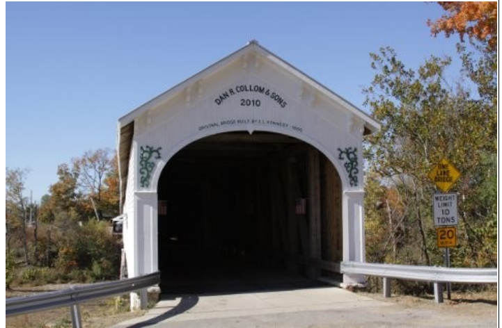
Rebuilt Moscow Bridge
